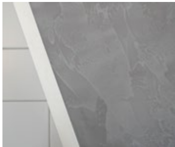
Substrate preparation for levelling on tiles with ARDEX R 4 RAPID and ARDEX R 1.
