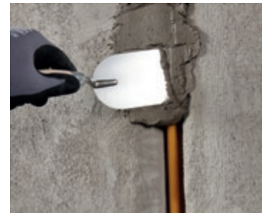
Suitable ground preparation for filling and leveling joints, break-outs and larger irregularities on plaster and concrete on larger depressions with ARDEX AM 70.
